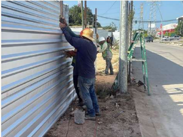
01 • Preliminary works and site enclosure
