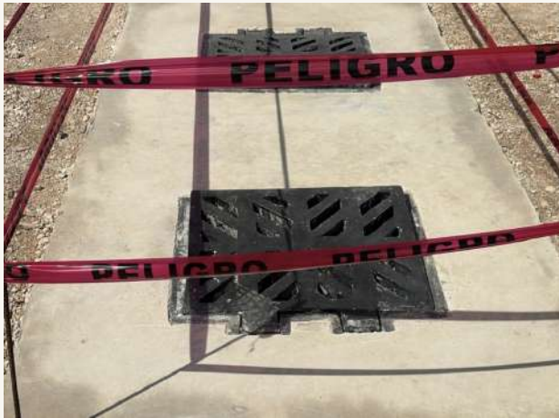
03 • Plumbing and storm drainage installations
