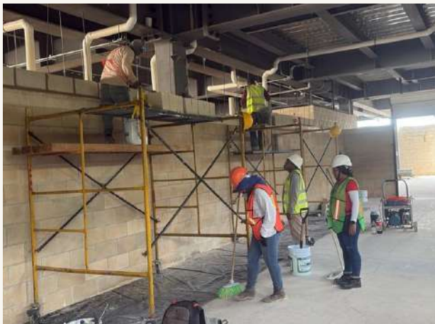
05 • Masonry and partitions
