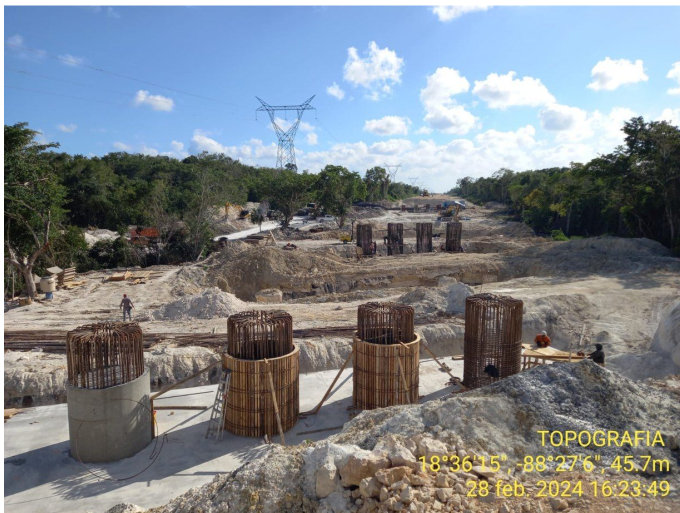
Deep foundations and concrete elements.
